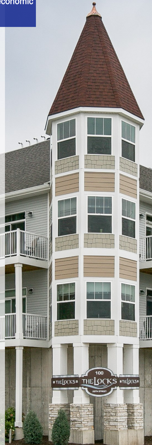
Transit-Oriented Housing The Locks 34 Residential Units // Rental New Construction
